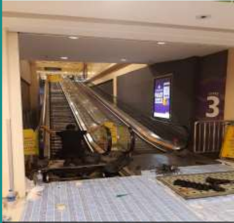
Replacement of traveller step chain and handrail
