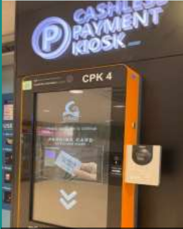
Upgrading of car park intercom
