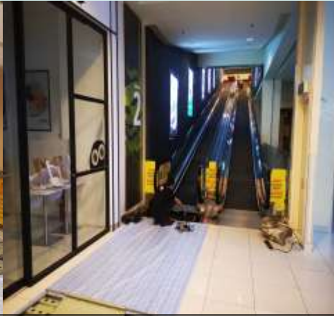
Replacement of traveller step chain and handrail
